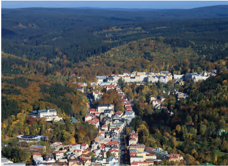
View north along Main Street, with its parallel expansive landscape of Central Park, to the principal spa quarter nestled in a sheltered E-W valley
